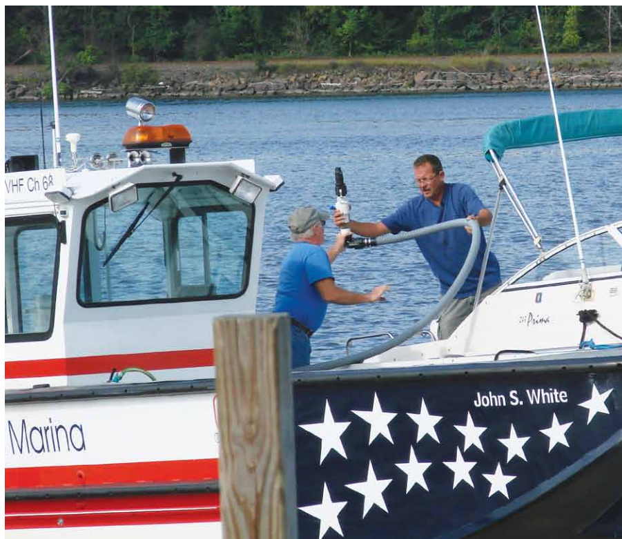
USING PUMP-OUT STATIONS to dispose of sewage from boats helps keep pollutants out of our waterways. Sewage collected by pumpout facilities is transported to on-land wastewater treatment plants.
